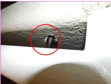
STAIRWAY to 2nd FLOOR Handrail Assembly
