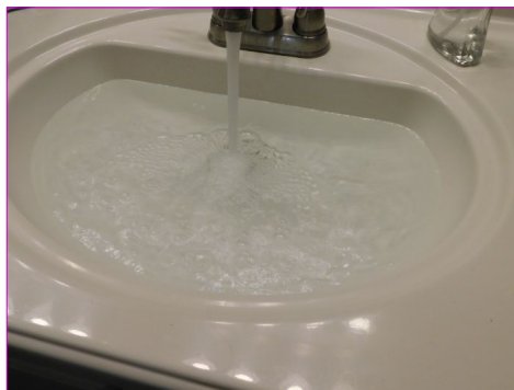
MAIN FLOOR HALL BATHROOM Single Sink
