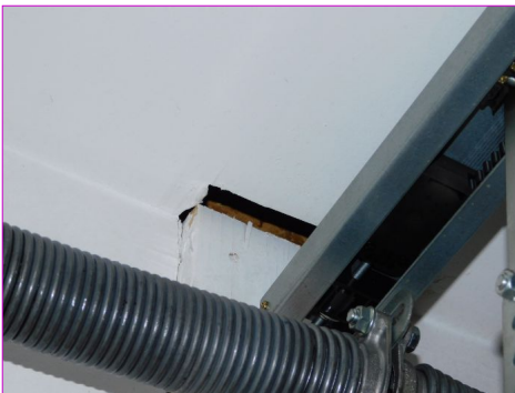
GARAGE Fire Separation
