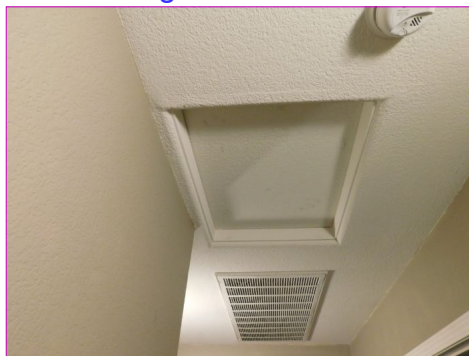
ATTIC Attic Access
