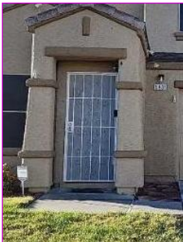
EXTERIOR VIEWS Front Entry
