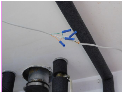
GARAGE Garage General Condition
