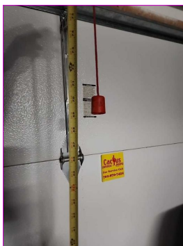
OVERHEAD GARAGE DOOR Manual Disconnect
