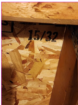
ROOF STRUCTURE EXTERIOR Sheathing
