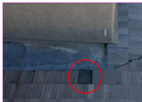
CONCRETE TILE ROOFS Tile Roof Condition
