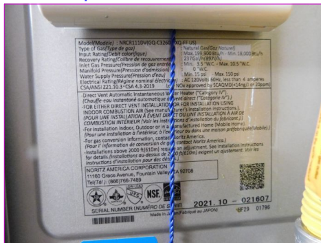
WATER HEATER Water Heater Data Plate Information
