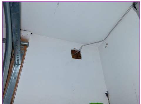
GARAGE Fire Separation
