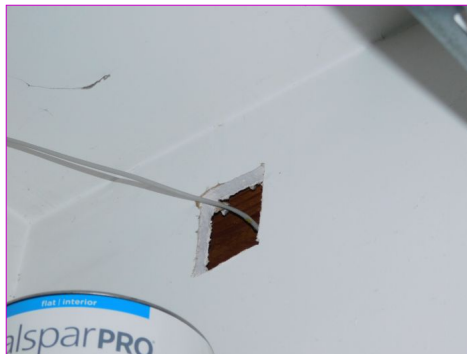
GARAGE Fire Separation
