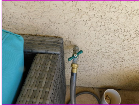
EXTERIOR PLUMBING Exterior Faucets
