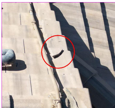
CONCRETE TILE ROOFS Tile Roof Condition
