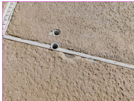
PATIO Patio Condition
