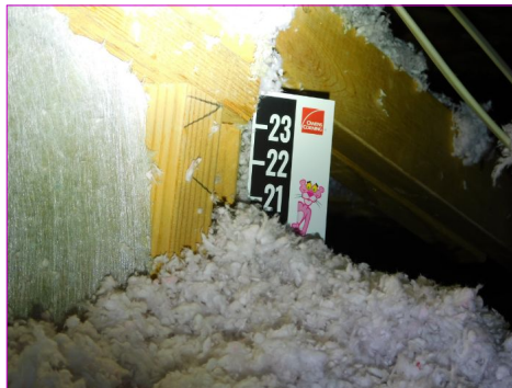
ATTIC Thermal Insulation Depth
