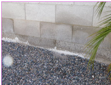
GROUNDS Boundary Walls
