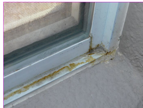
WINDOWS Window Sill/Jamb Condition
