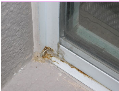
WINDOWS Window Sill/Jamb Condition
