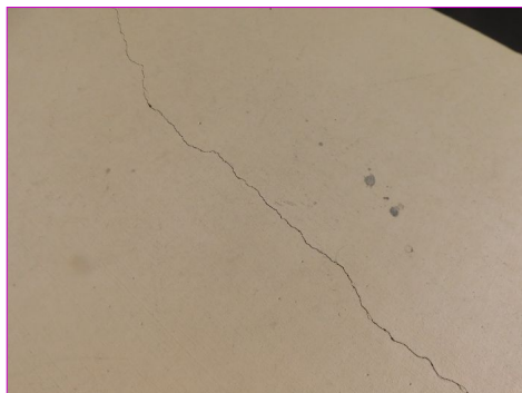
PATIO Patio Slab Condition
