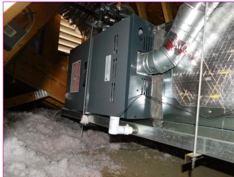
FURNACE General Condition
