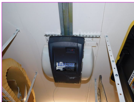
OVERHEAD GARAGE DOOR Automatic Opener
