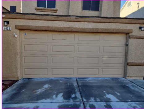
OVERHEAD GARAGE DOOR General Condition
