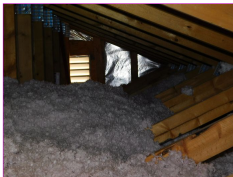
ATTIC Thermal Insulation Condition
