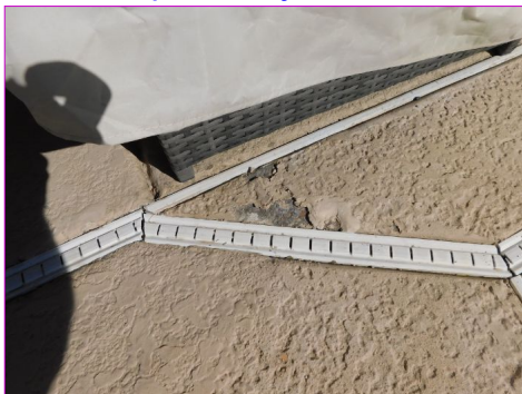
PATIO Patio Condition
