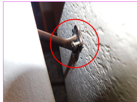
STAIRWAY to 2nd FLOOR Handrail Assembly
