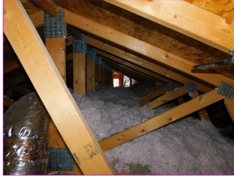
ATTIC Thermal Insulation Type
