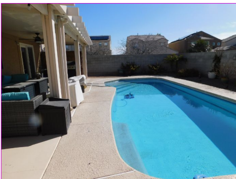
SAFETY HAZARDS Pool Barriers
