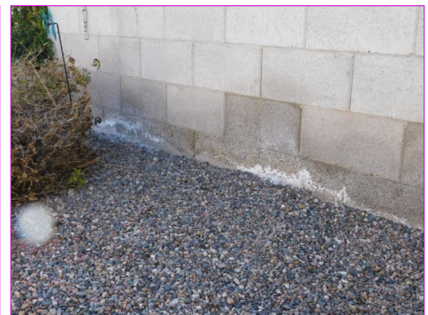
GROUNDS Boundary Walls
